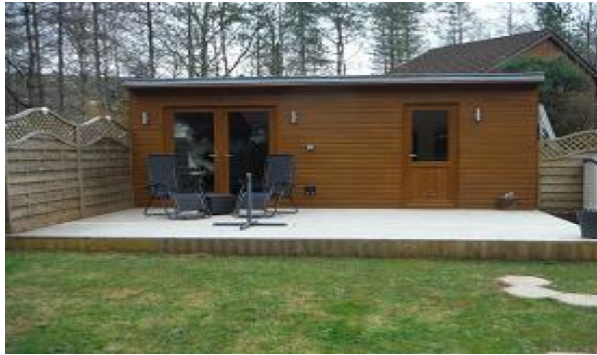
View of building as seen from the applicants garden.
